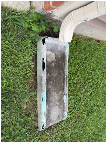
Front right side downspout replace extension
