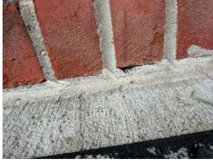
Under front door
