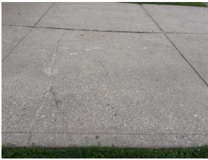
Cracked and sunken piece poured concrete seems to have been repaired previously
