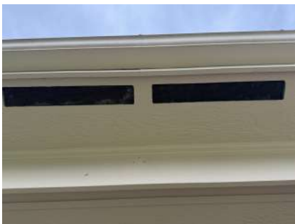
Front porch soffits
