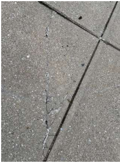
Cracked and sunken piece poured concrete seems to have been repaired previously
